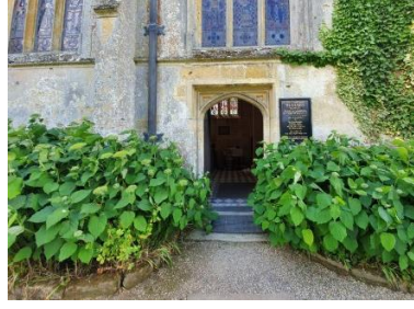
Ramped access into Church
