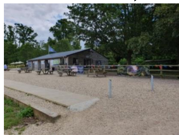
Sloped access from car park to Visitor Centre
