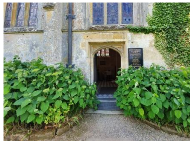
Ramped access into Church
