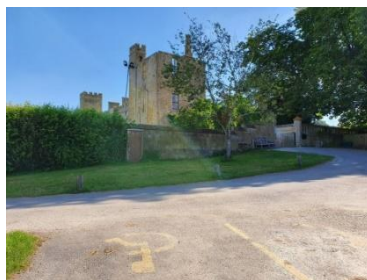
Castle Terrace accessible parking bays
