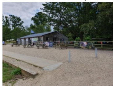
Sloped access from car park to Visitor Centre
