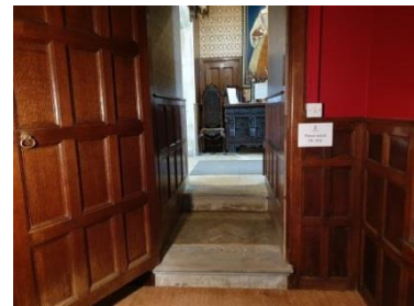
Stepped access to South Hall via Knot Corridor
