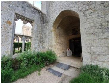
Ramped access to South Hall – entrance lobby to castle rooms
