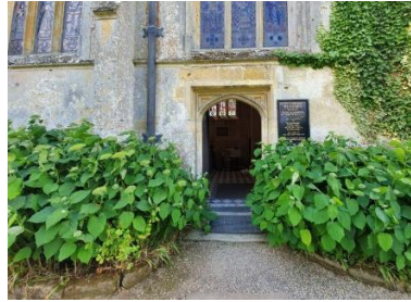
Ramped access into Church
